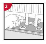
Drill holes 18mm/ ¾" larger than the diameter of the pipes. Cut out the floorboard (with the thinnest blade possible). Install the floorboard, glue the cut out piece back in place.
